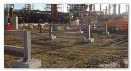
Cyntech redesigned and installed all the foundations (150 in total) using screw piles with concrete pile caps. The client realized significant savings in both cost and time.
