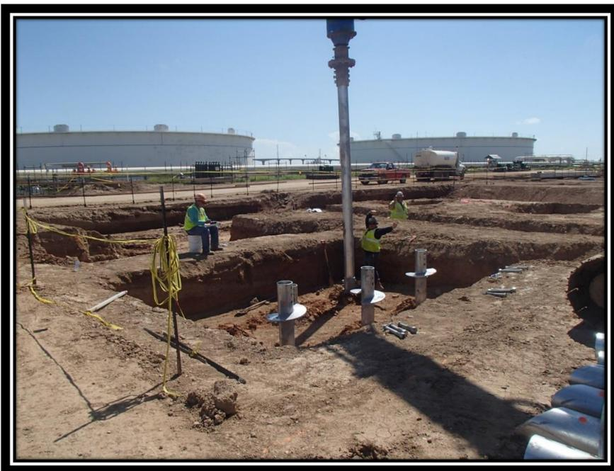
Typical Helical Pile Foundation
