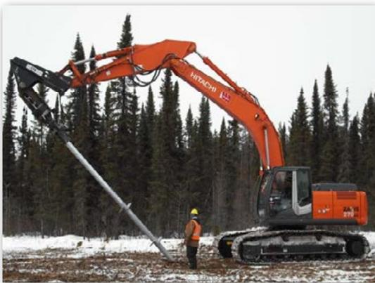
Manitoba Hydro was constructing a new double circuit 230kV power transmission line in northern Manitoba. New towers needed to be erected, and the soil conditions required an innovative solution. Cyntech was able to provide foundations for these towers, at considerable savings over traditional methods. In all, Cyntech provided 1,040 guy anchors and 260 foundation piles to support the towers.
