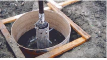
Helical pile installation.
