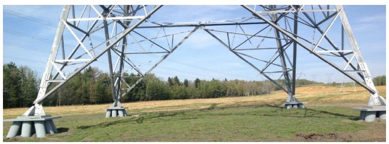
Cyntech designed and supplied helical piles for 137 lattice tower structures.
