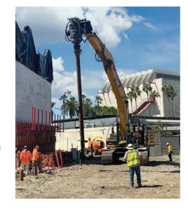
today—a faster, lower-cost, more efficient high-capacity deep foundation technique that provides significant load capacity (greater than 1,000 kips or 4500 kN) with less impact to your z and the environment.
