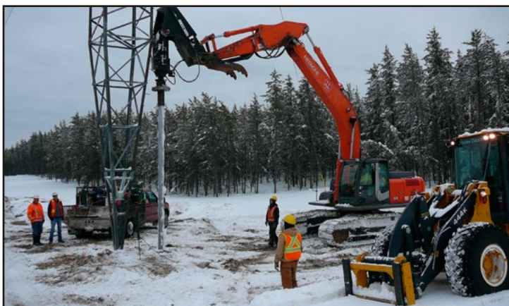
FOUNDATION REPAIR – ELECTRICAL TRANSMISSION TOWER
