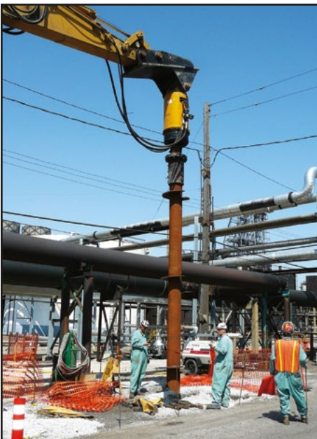
CONGESTED AREA INSTALLATION
